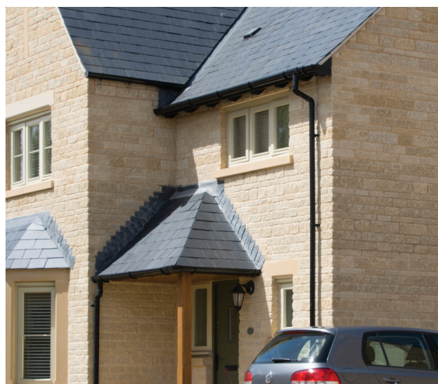
Sized to course using three sizes of Oolite.
